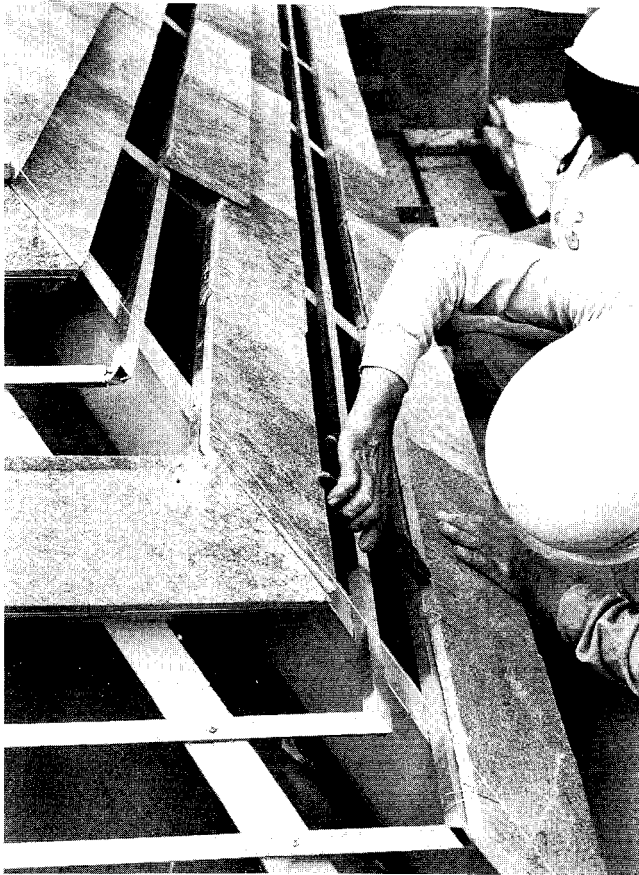
Fig. 5. Installing tepei stone at the Tanpopo House.
